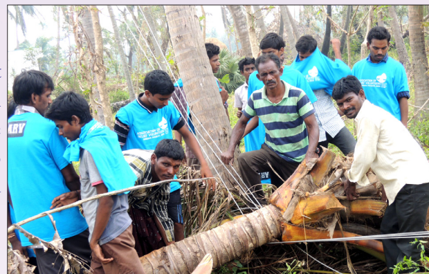
ARV Volunteers removing fallen tree to restore Electricity
